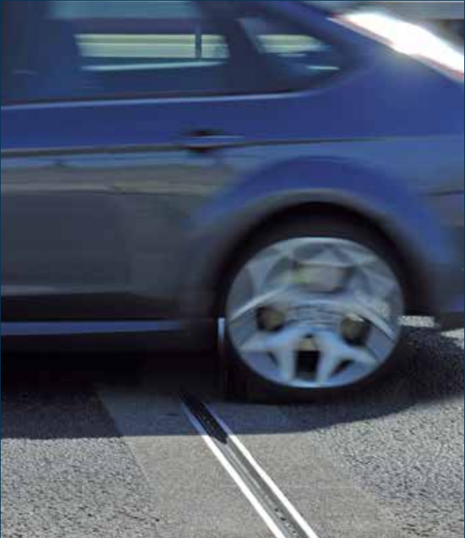
A close up of the BEJ expansion joint system not normally seen by the travelling public.
